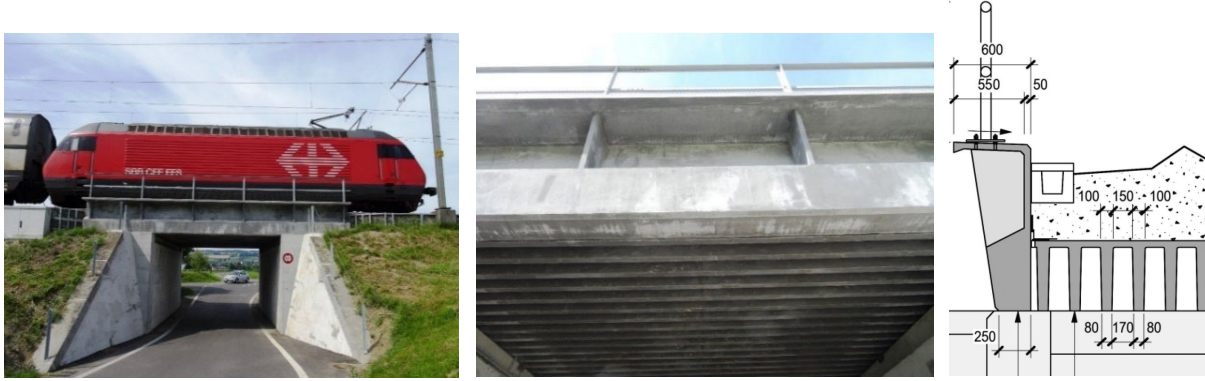
Figure 4: Short span, ribbed slab UHPFRC railway bridge
