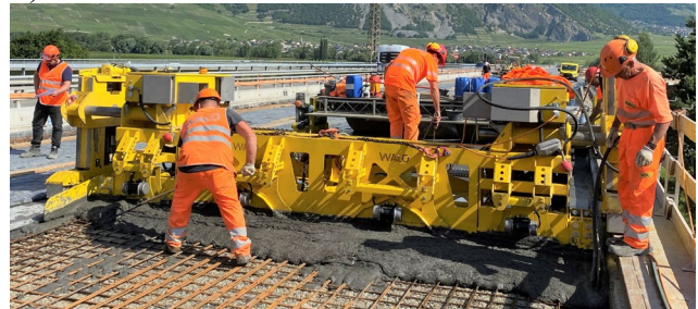
Figure 1: (a) cross section of a box girder and fatigue-prone domains, (b) casting of R-UHPFRC on top of the slab of the box girder of a road bridge.
